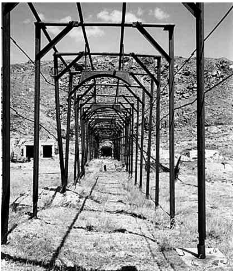
Figure 30. View of a structure at tunnel 169/2 constructed to hold a gas-filled bag used in a radiation effects experiment. In this test, radiation was directed out two diverging tunnels from a centrally-located device.
